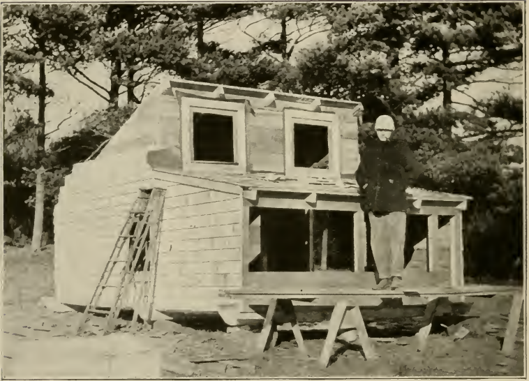
Building a portable colony type Woods' open-air poultry house, 10x16 ft., Wozelma Farms Producing Company, Silver Lake, Mass.
