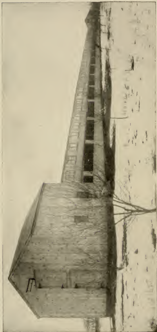
View of F. M. Peasley's fresh-air poultry house, Cheshire, Conn. An open-front house built to accommodate 2,000 layers. Adapted from plans of semi-monitor-top open-front poultry house designed by Dr. P. T. Woods. This mammoth house has "proved entirely satisfactory."
