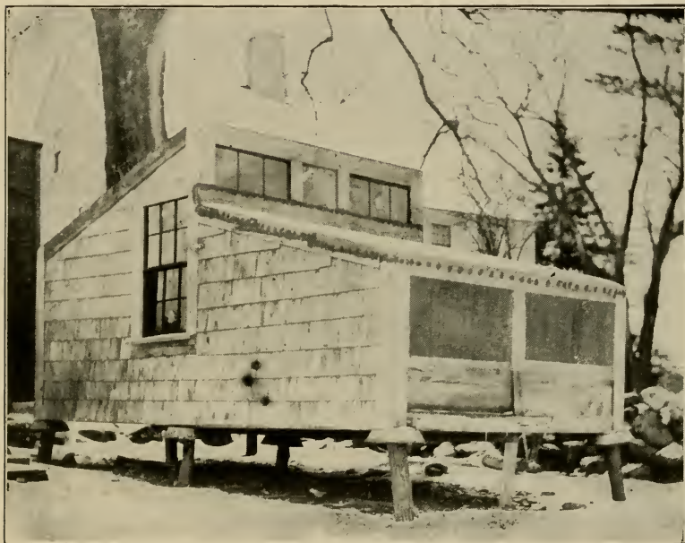
Experimental Woods' Open-air House built in 1908 at Topsfield, Mass. This house has a double board floor and is set on posts over which large pans have been inverted to make the house rat proof. View shows south front and west side. (Photo by Dr. Woods.)
