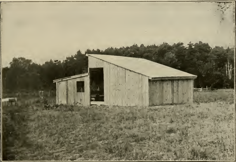
DR. P. T. WOODS' IMPROVED OPEN-AIR POULTRY HOUSE. Fig. 10.—View of east and north end before putting on roofing. Opening shown for door and window. (Photo by Dr. Woods.)
