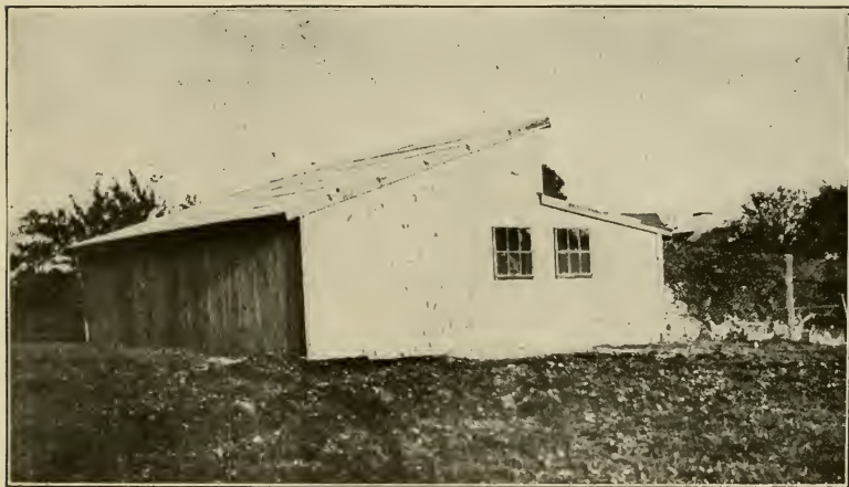
View of north and west sides of Dr. P. T. Woods' Improved Open-air Poultry House as completed and ready for painting. Roof is covered with Amatite. (Photo by Dr. Woods.)
