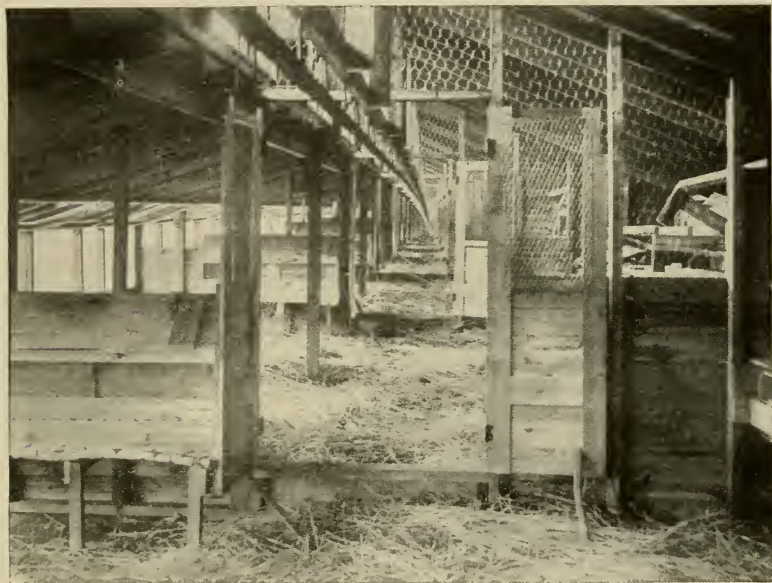
Interior view of F. M. Peasley's fresh-air house for 2,000 layers, Cheshire, Conn. Shows arrangement of track for feed car, hoppers, roosts, partitions, etc. (See page 64.)
