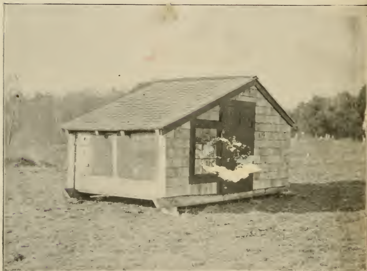
Portable Tolman pattern open-front house, 6 ft. wide by 10 ft. deep, built on skids. Used for small chicks by Wozelma Farms Producing Company, Silver Lake, Mass. (Photo by John E. Zeller.)
